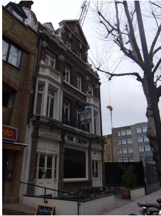
The Crown Public House, Blackfriars Road
